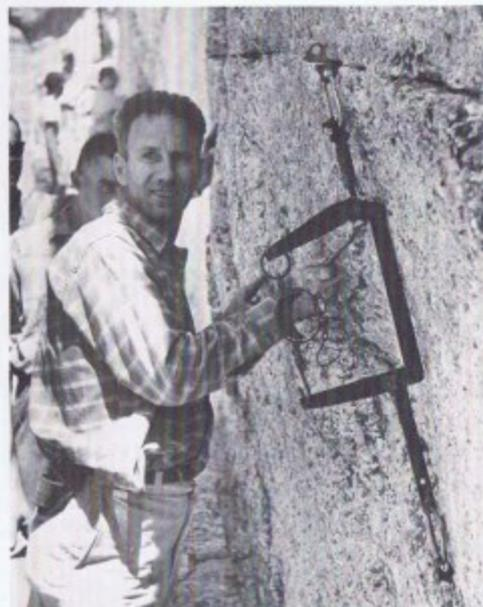
Chuck Wilts with a primitive piton-testing rig.
